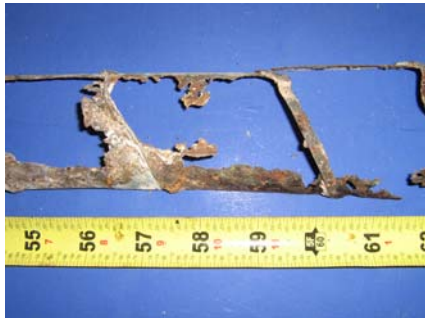
Top of South Duct
