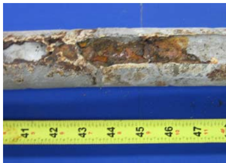
South Duct Grout
