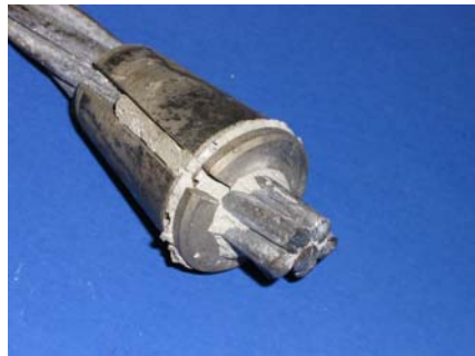
South Duct Strand with Wedges
