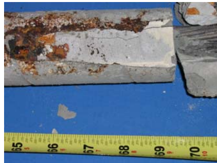
North Duct Grout
