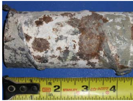
Top of North Duct
