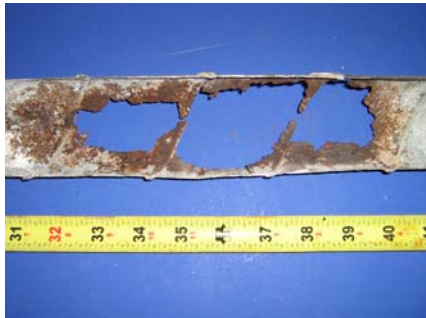
Top of North Duct
