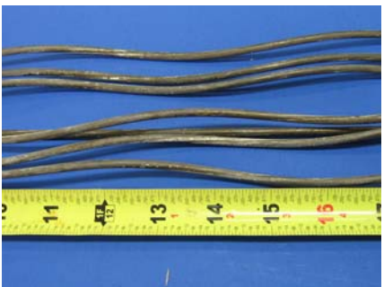
South Duct Strand
