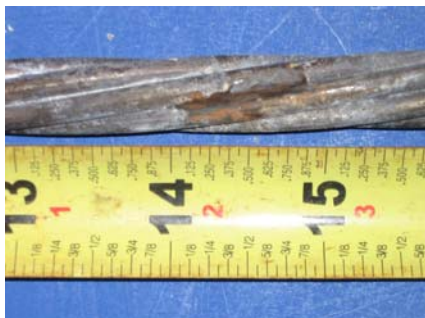
South Duct Strand
