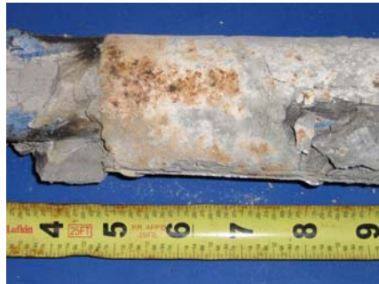
North Duct Grout
