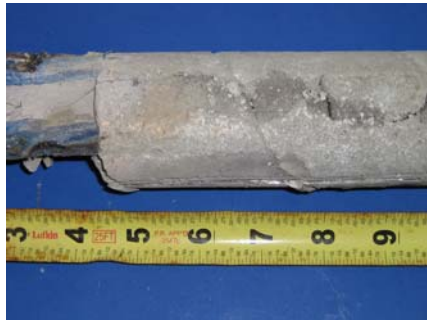
South Duct Grout
