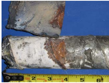
Top of South Duct
