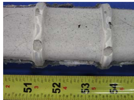
North Duct Grout
