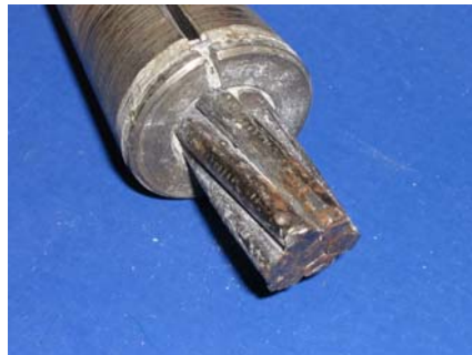
North Duct Strand With Wedges
