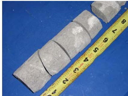
North Duct Grout
