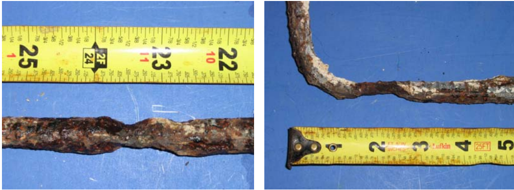
Figure 5.22: Beam 1.2 Autopsy Elements-Longitudinal Bar (Left) and Stirrup (Right)
