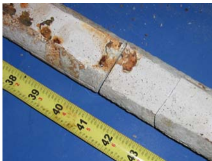
South Duct Grout
