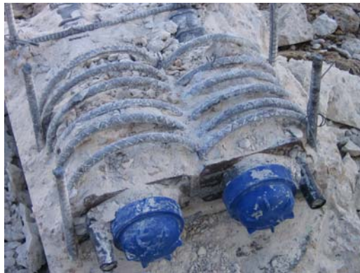
Figure 5.12: Removal of Post-Tensioning Anchorages (East End Anchorage of Beam 2.12 pictured)
