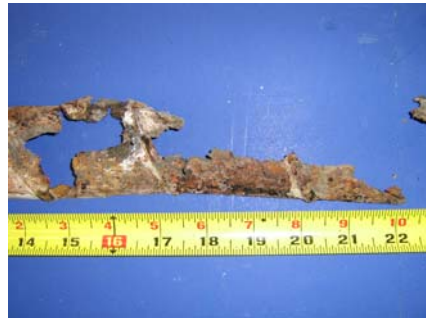
Top of North Duct
