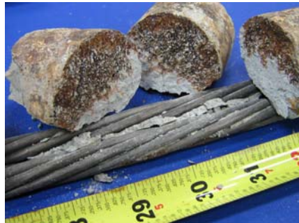
North Duct Grout
