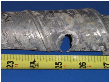
Top of North Duct
