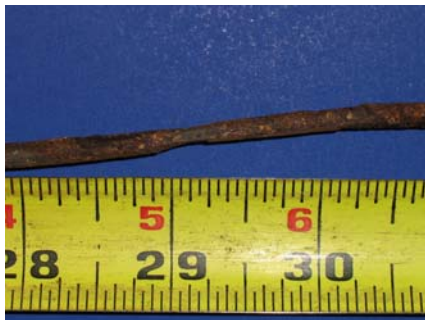
Single Wire from South Duct Strand
