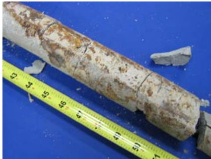
South Duct Grout
