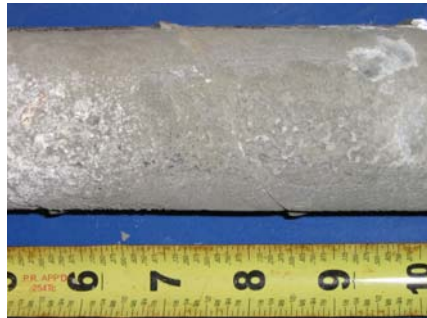
North Duct Grout
