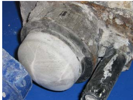
South Duct Grout Cap
