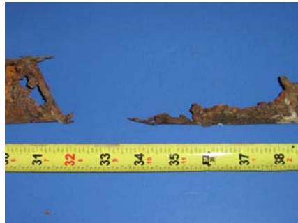
Top of North Duct
