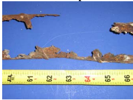
Top of North Duct
