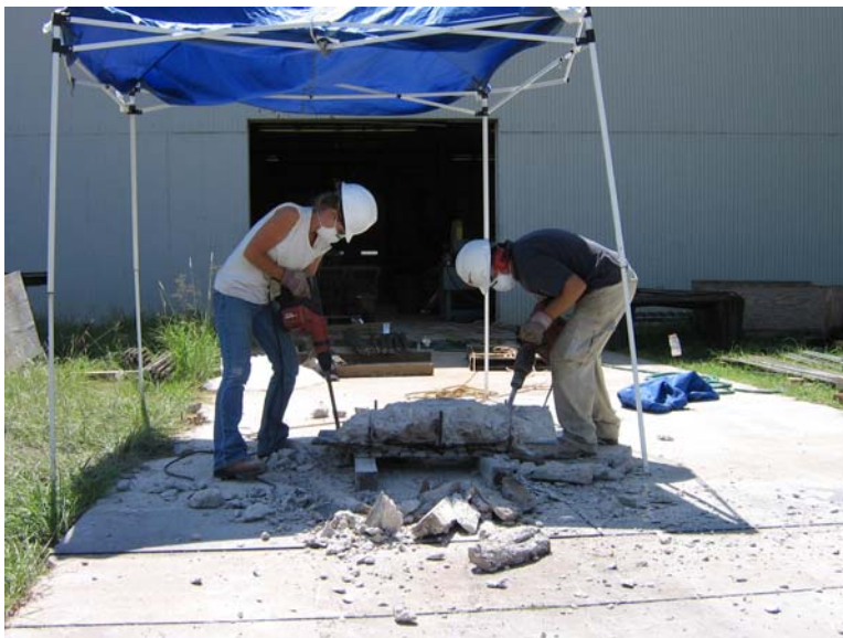
Figure 5.9: Breaking up of Block (Phase I Beam 1.1 Pictured)
