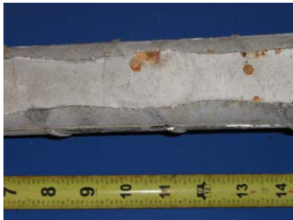
South Duct Grout
