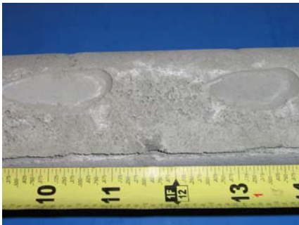
North Duct Grout
