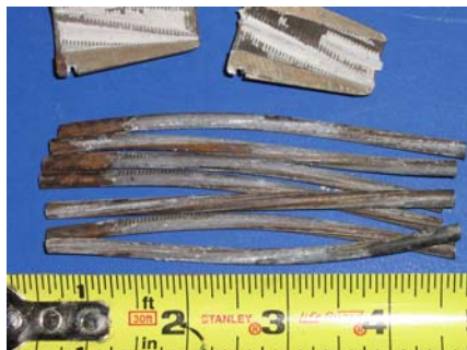
South Duct Strand
