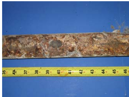
North Duct Grout
