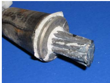
North Duct Strand With Wedges
