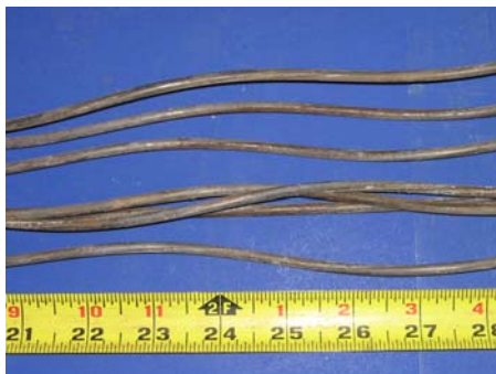
South Duct Strand
