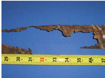
Top of South Duct
