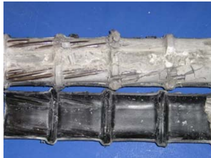
North Duct Grout (From Bottom)
