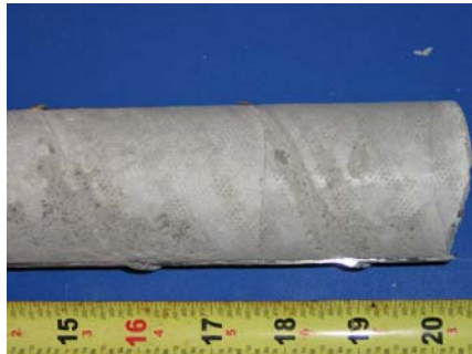
South Duct Grout
