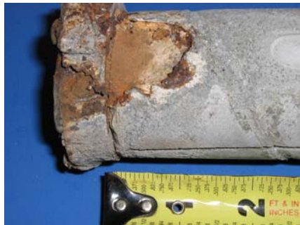
South Duct Grout
