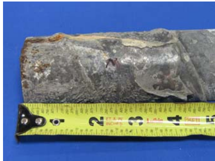
Top of South Duct
