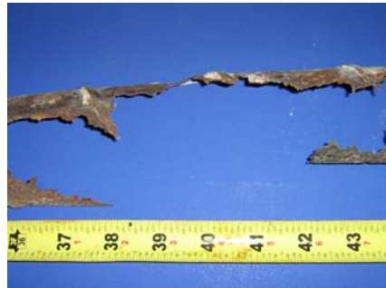
Top of North Duct
