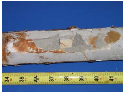
North Duct Grout
