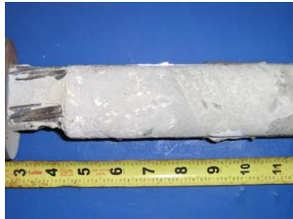
North Duct Grout
