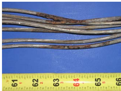
South Duct Strand
