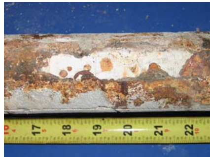
North Duct Grout
