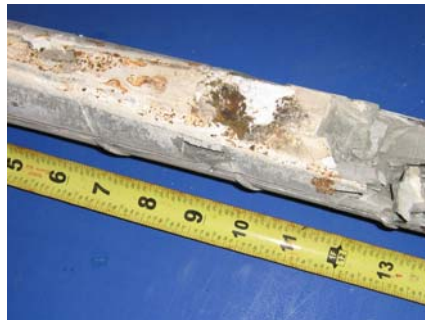
North Duct Grout
