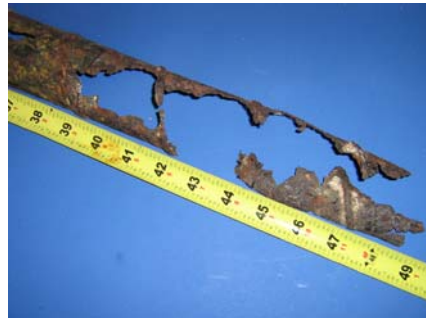
Top of North Duct
