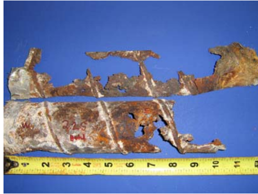
Figure 5.35: Beam 2.2 South Duct Splice
