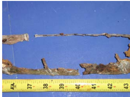
Top of North Duct
