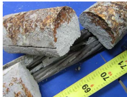
North Duct Grout
