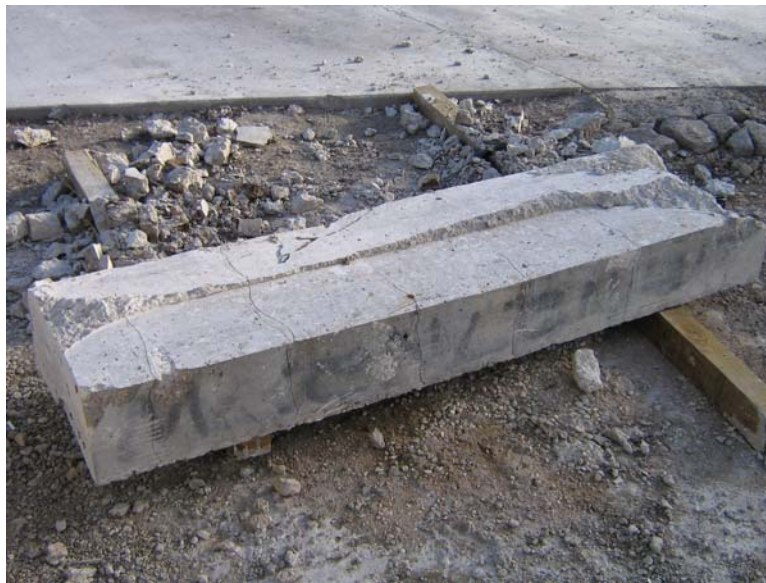
Figure 5.7: Typical Center Block Removed from Beams (Phase II Beam 2.7 Shown)
