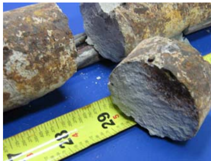
South Duct Grout
