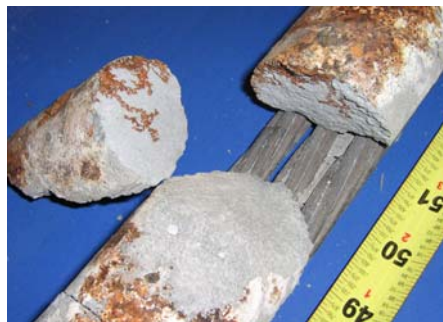
North Duct Grout
