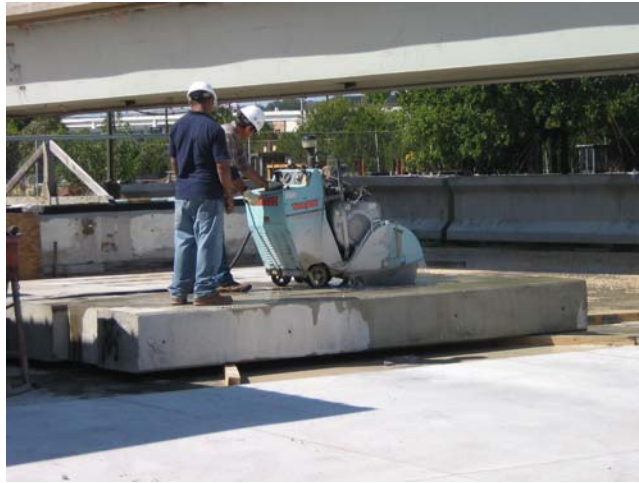
Figure 5.6: Cutting of Beams (Phase I Beams Pictured)
