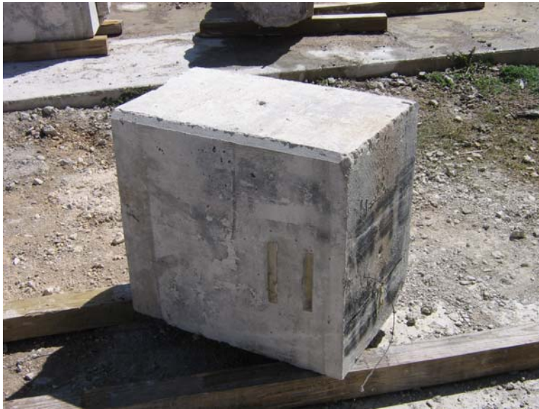
Figure 5.8: Typical End Anchorage Block Removed from Phase II beams 2.7, 2.9, and 2.12 (Beam 2.12 East End Shown)
