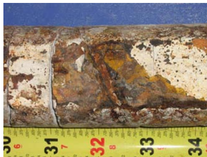
North Duct Grout
