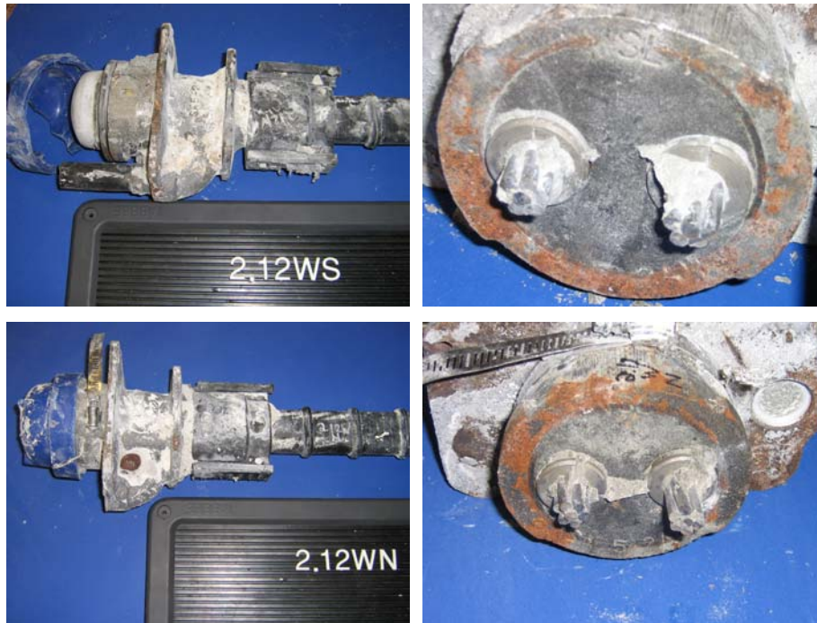
Figure 5.108: Beam 2.12 West End Anchorages (Control End)-South Duct Anchorage (Top, Left and Right) and North Duct Anchorage (Bottom, Left and Right)
