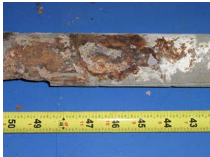
South Duct Grout
