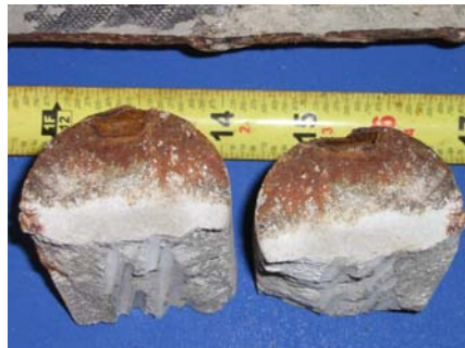
South Duct Grout
