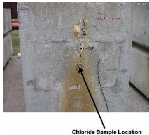
Figure 3.7: Chloride Sample Location for Anchorage Exposure Specimens
