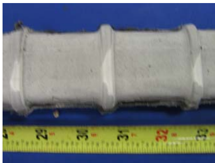
South Duct Grout
