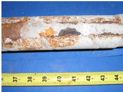
South Duct Grout
