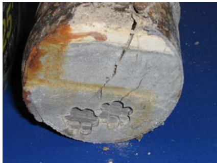
South Duct Grout
