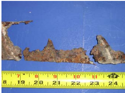
Top of South Duct
