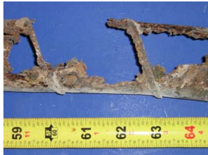
Top of North Duct
