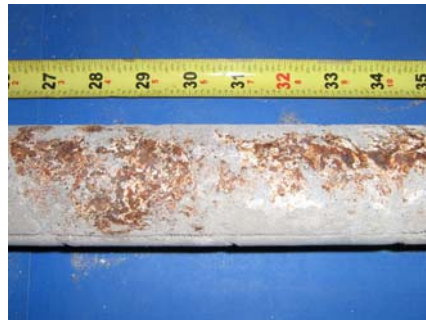
North Duct Grout
