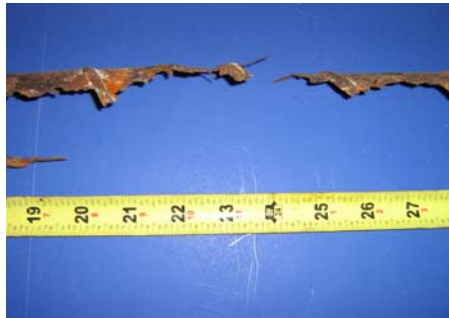
Top of South Duct
