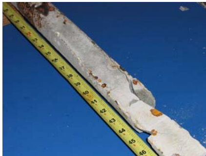
South Duct Grout
