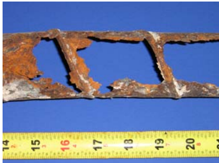
Top of South Duct
