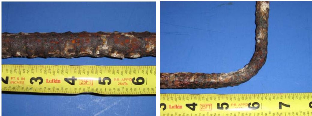
Figure 5.17: Beam 1.1 Autopsy Elements-Longitudinal Bar (Left) and Stirrup (Right)
